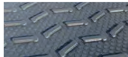
rib profile on the surface
